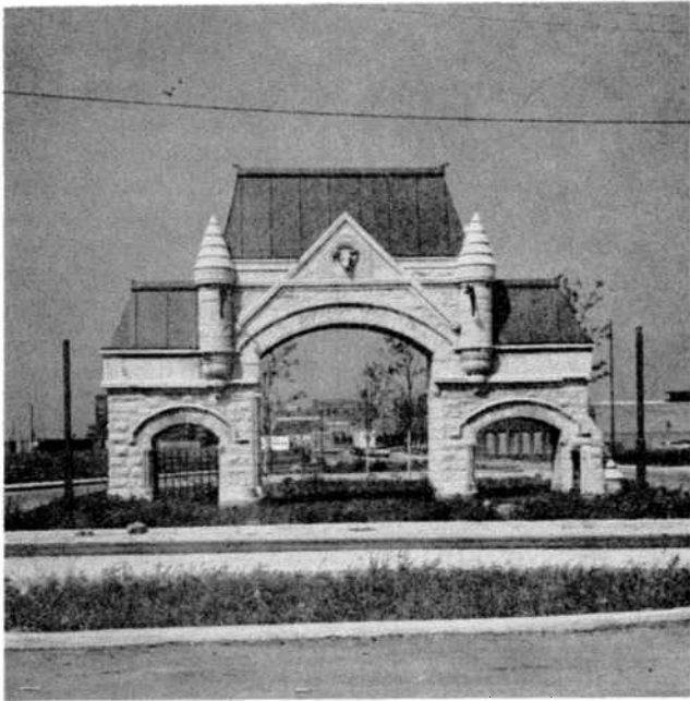
The restored gate with site work partially complete. Trees have been planted, lamp posts installed, and eventually all ground not landscaped will be inset with paving bricks saved from the pen area. (Barbara Crane, photographer)
